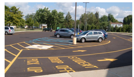
Parking lot re-pavement at Susick Elementary.
