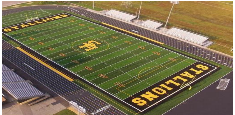
A running track, football field turf and stadium sound system were installed at Sterling Heights HS.
